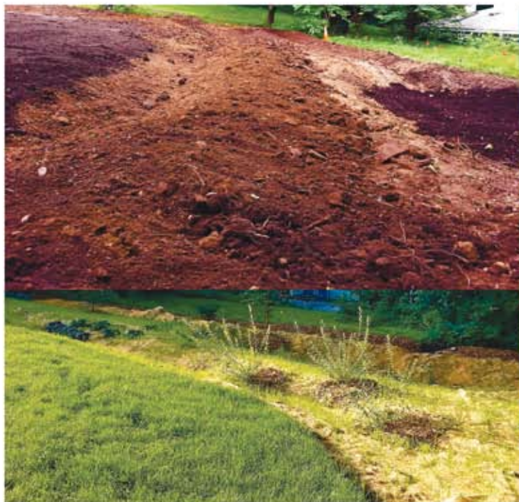
Top: Reshaping the lot to channel water. Below: Two weeks after seeding.
